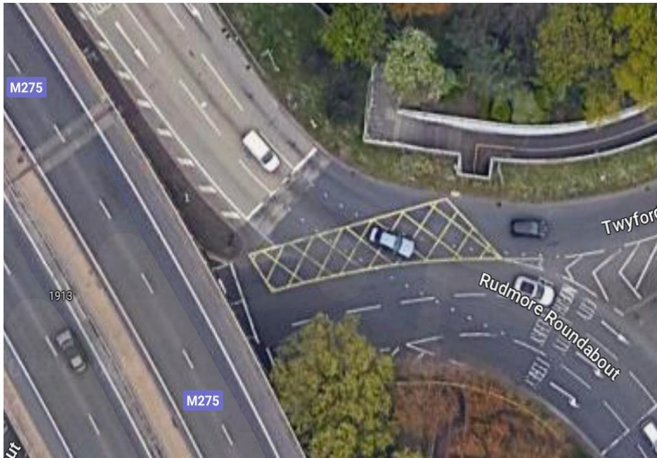
Rudmore Roundabout/M275 slip- Box junction
